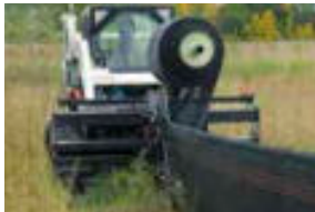
Silt Fence Installer P. 148
