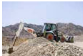
Bucket, Digging P. 341
